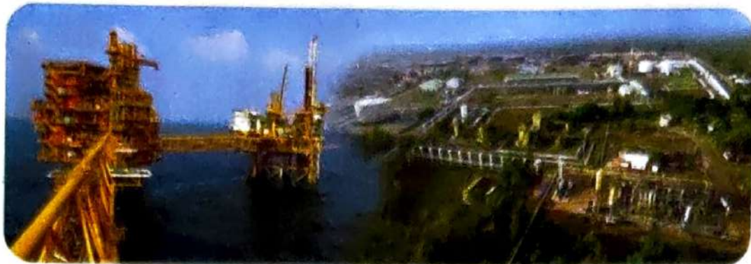
Offshore Platform, HPHT Asset
